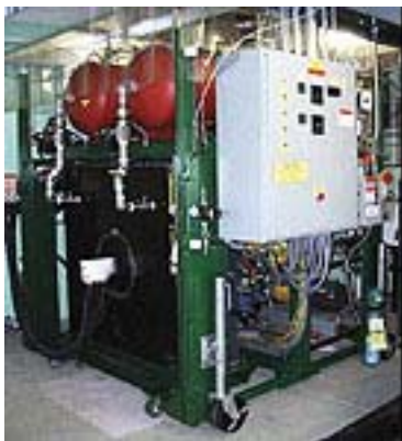
Fig 4-2. GE Electrolyzer – “$3/kg” (hydrogen production cost)
